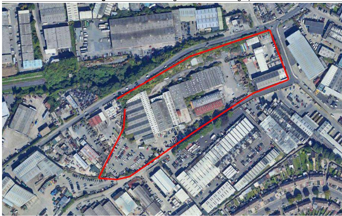
Figure 16.1 Existing Site Aerial Photograph
