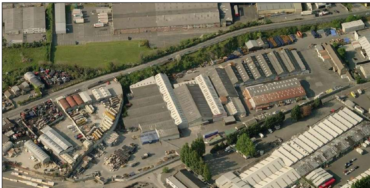
Figure 15.7 Aerial View of Site and Immediate Environs – from south
